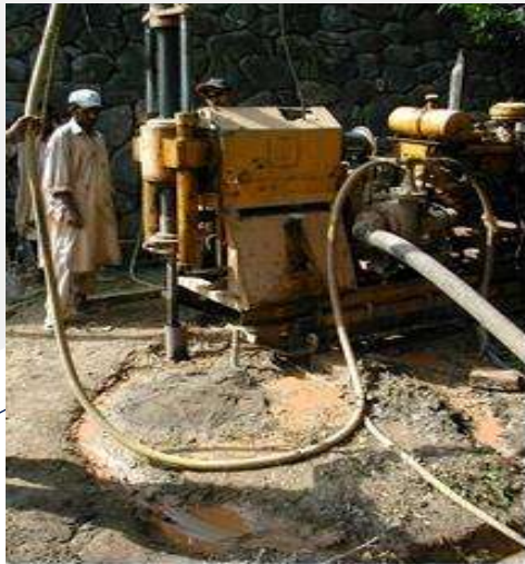
Geotech Soil Investigation
